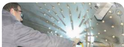
Installation of Shoulder Studs
